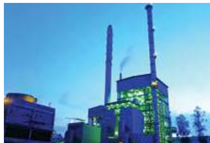
NPS Double A Power Plant 2
