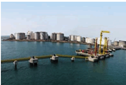
SCG Rayong Tank Terminal
