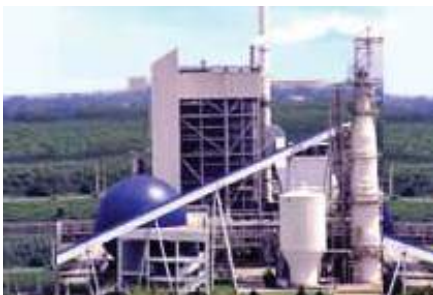
NPS Double A Power Plant
